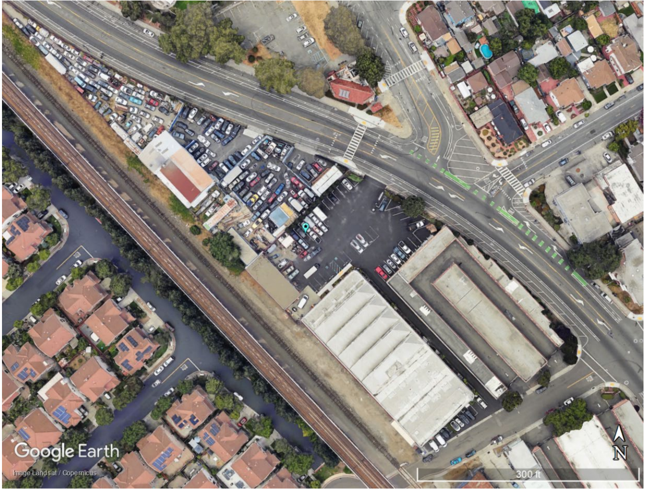
Image to show distance to surrounding buildings
