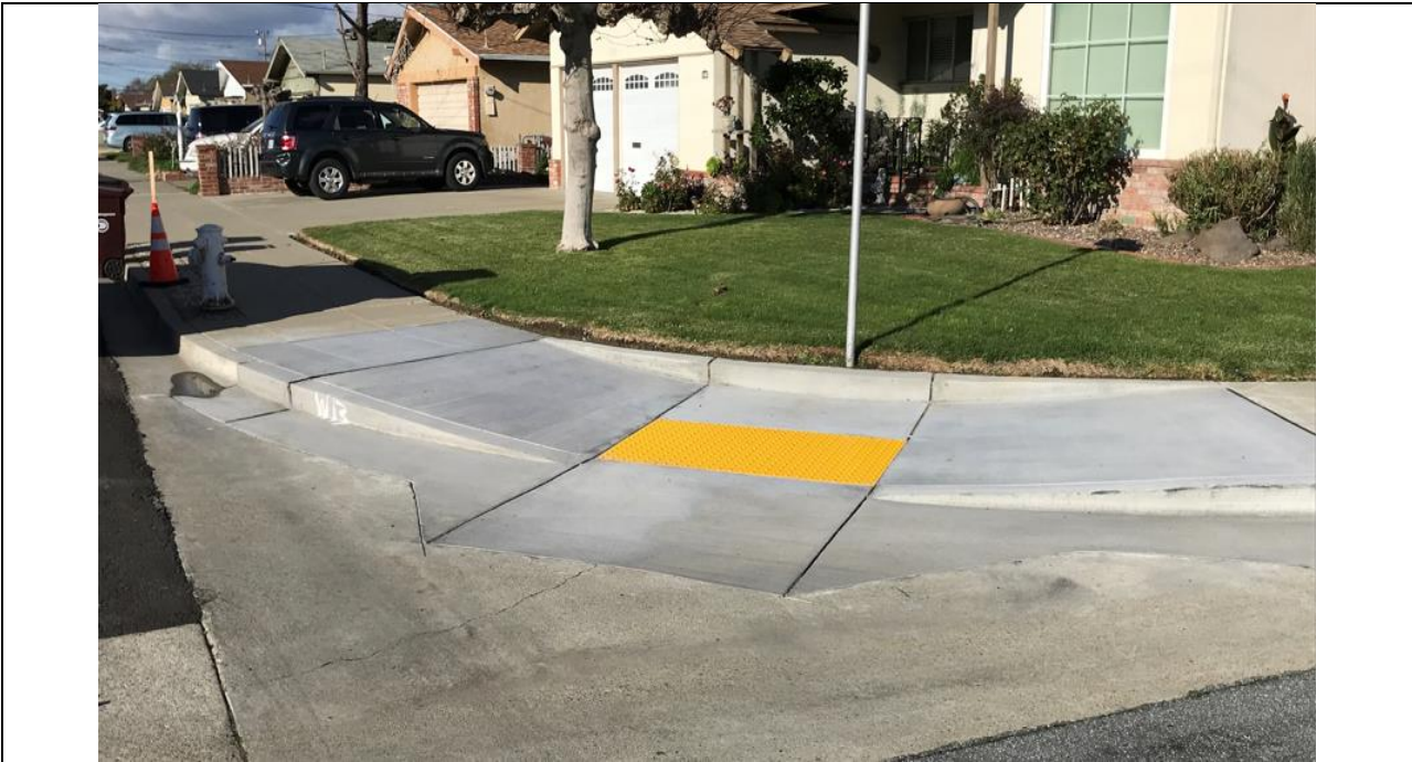
COMPLETED ACCESSIBLE CURB RAMP
