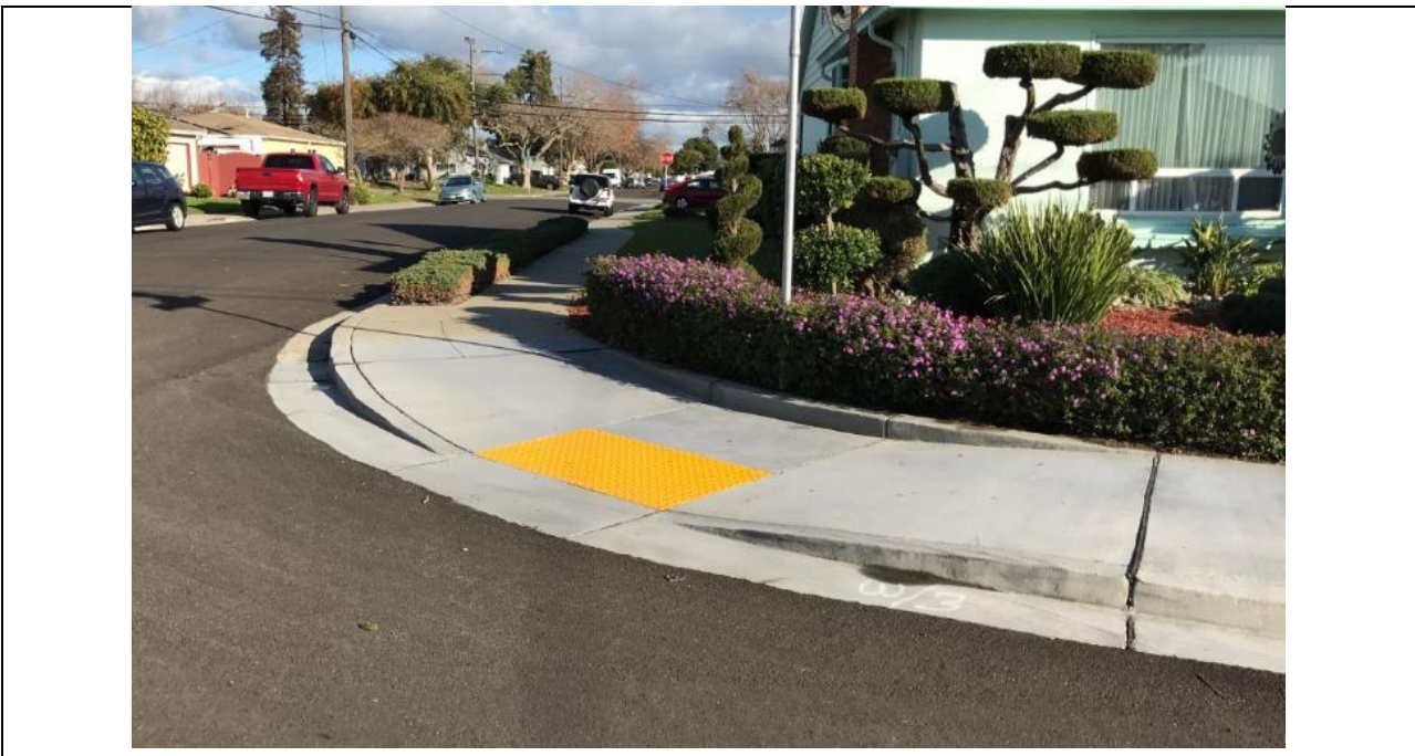
COMPLETED ACCESSIBLE CURB RAMP
