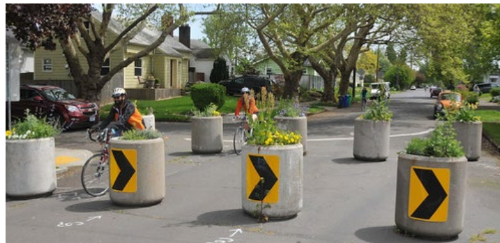
Figure 23 Example of Traffic Diverter
