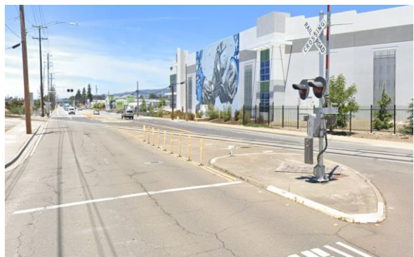
Railroad crossing locations often have gaps in pedestrian and bicycle facilities.
