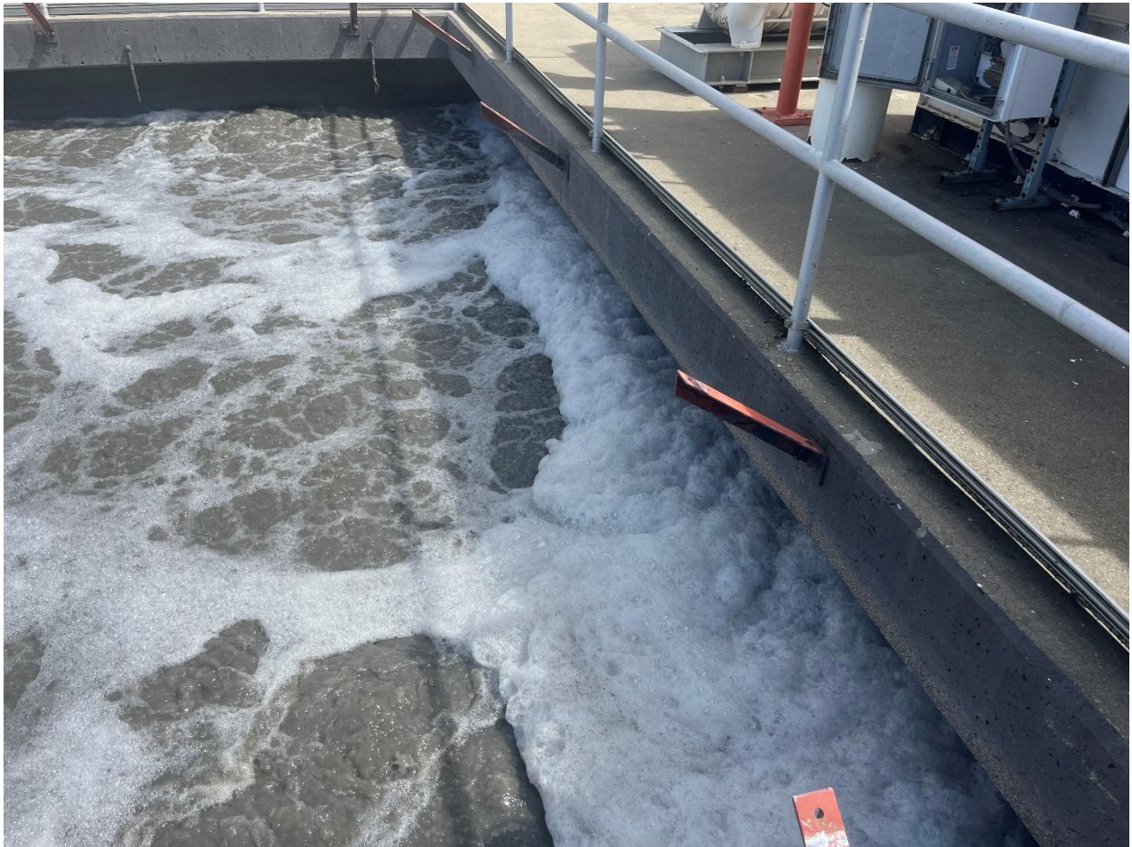
Figure 4-12. White Foam Formation in the Aeration Basins during the 2025 Plant Upset
