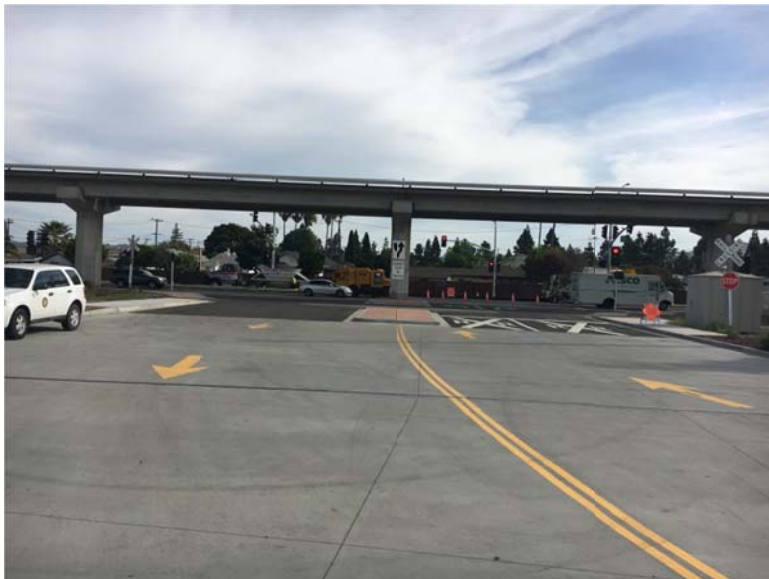
Widened Polar Way - Looking East
