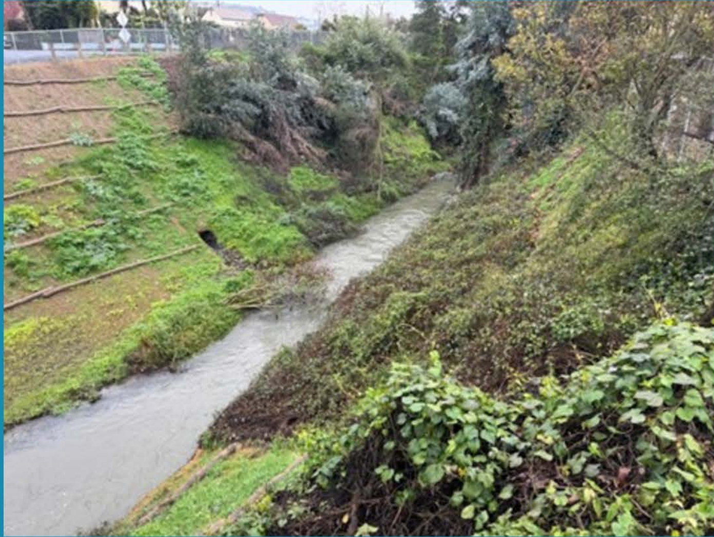
Cary/Haas Pedestrian Bridge Replacement
