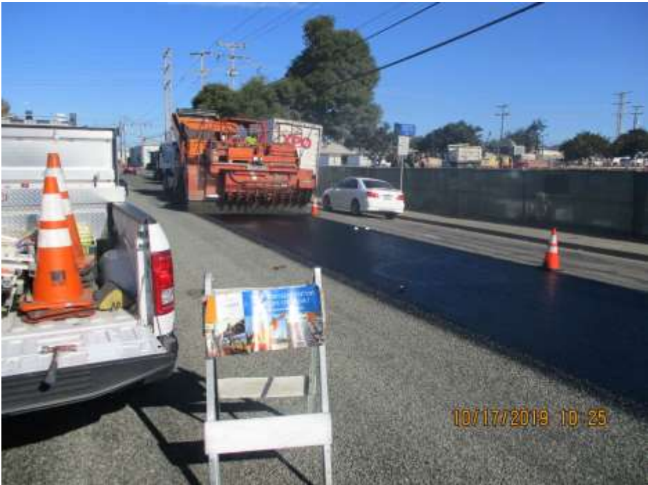
Street sealing in progress
