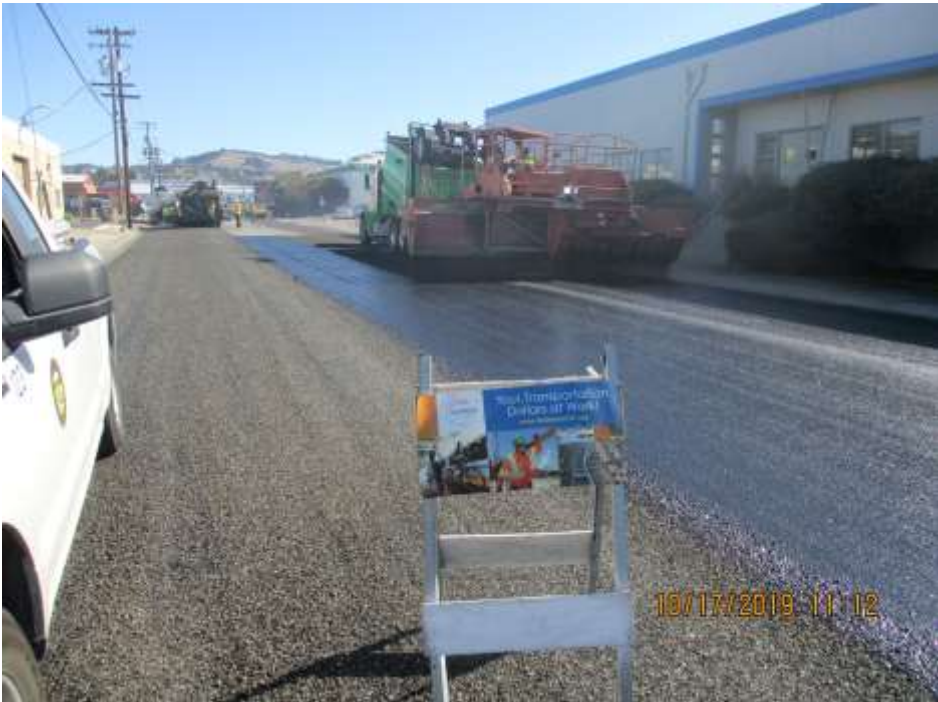
Street sealing in progress
