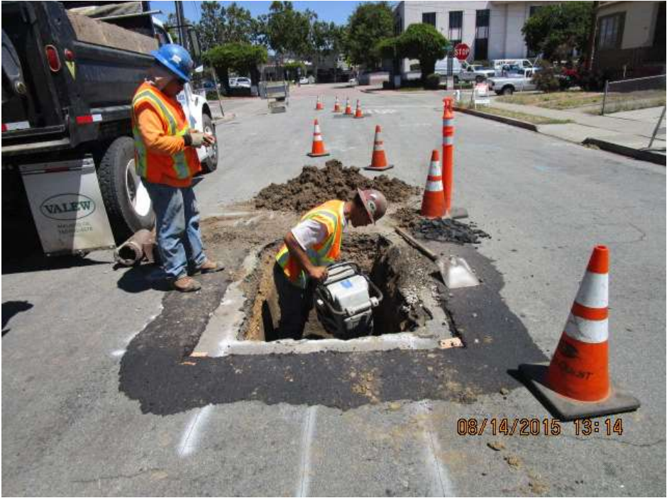
Sanitary sewer pipe repair
