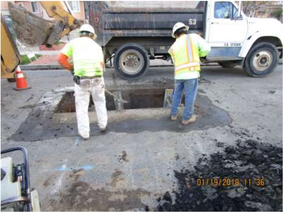
Sanitary sewer pipe repair
