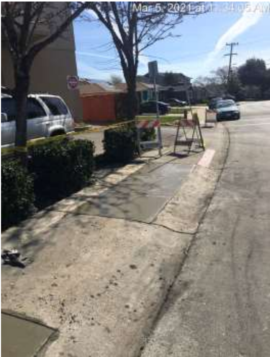
Sidewalk repair in progress
