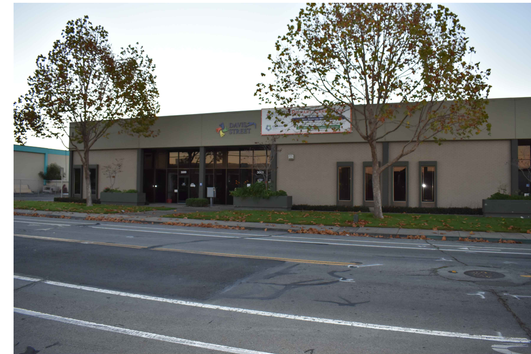
EXISTING PHOTO LOOKING SOUTH-EAST
