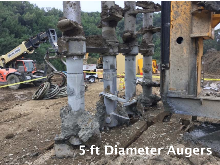
Seepage Trench and CDSM Buttress
