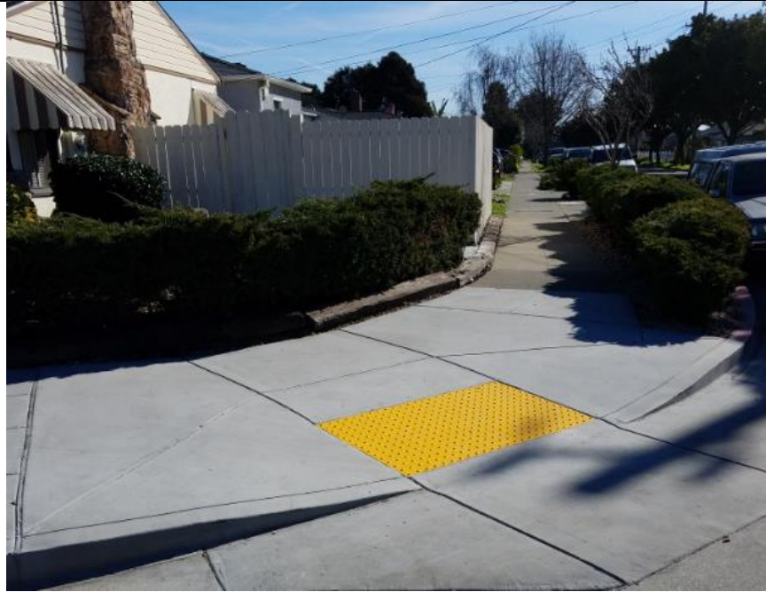
COMPLETED ACCESSIBLE CURB RAMP
