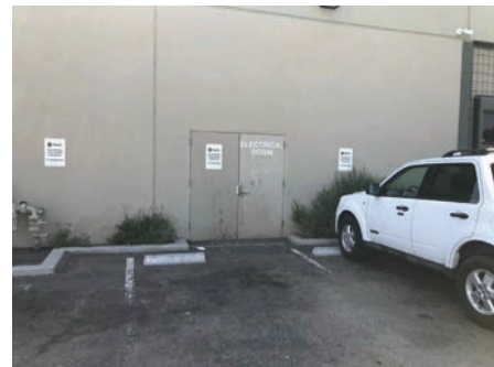
⑦ ELECTRIC CLOSET
