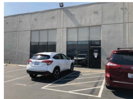
⑬ REAR ENTRANCE OF 3081 TEAGARDEN STREET
