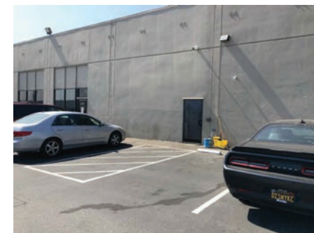
⑭ REAR ENTRANCE OF 3089 TEAGARDEN STREET
