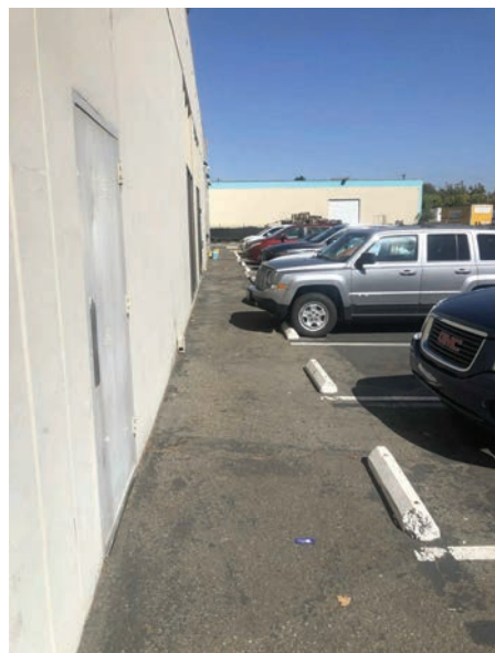
⑪ REAR ENTRANCE OF 3081 TEAGARDEN STREET
