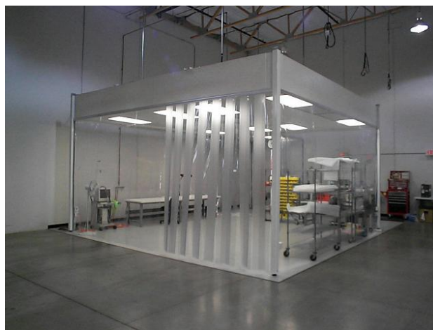
Figure 4. Modular Clean Room
