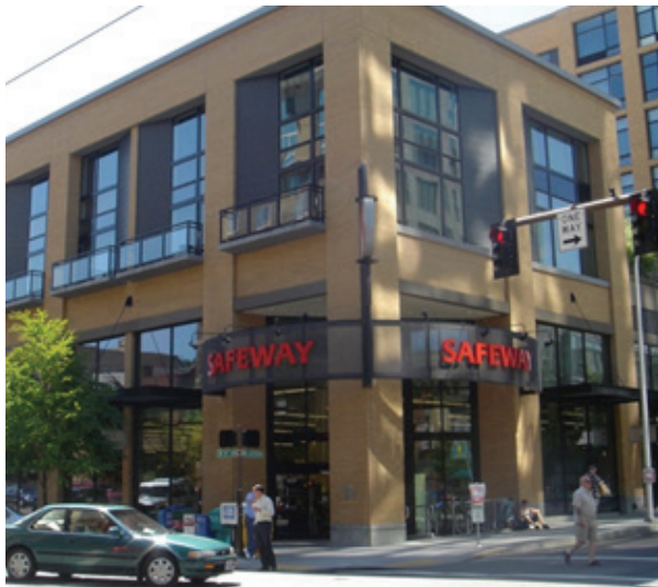
Example of ground-floor transparency and corner entry facing both streets in an active ground-floor retail use
