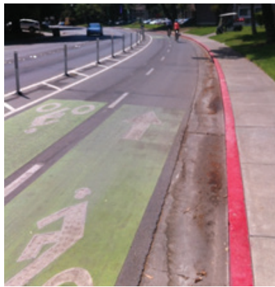
Example of two-way Class IV separated bikeway
