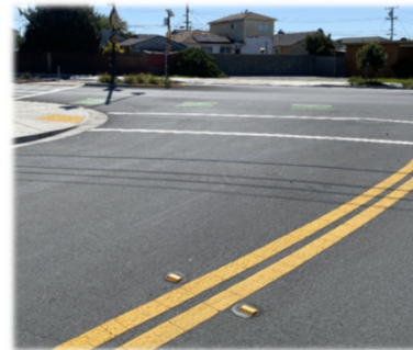
Pavement Surface Seal
