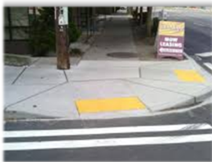
Accessible Curb Ramps
