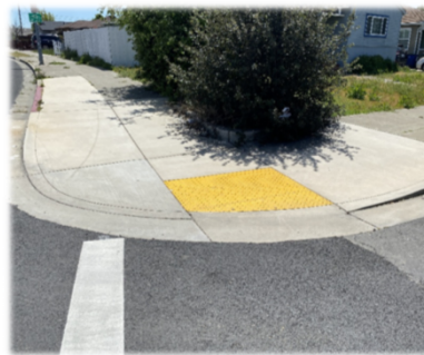
Tighten Turn Radii at Corners
