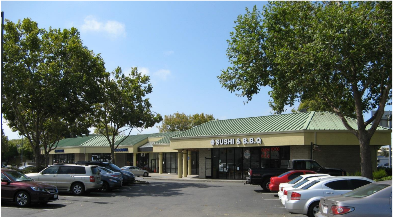
Buildings on triangular site at corner of Washington Avenue and Lewelling Boulevard, originally part of PD-83-3 but now under separate ownership and not included in proposed project
