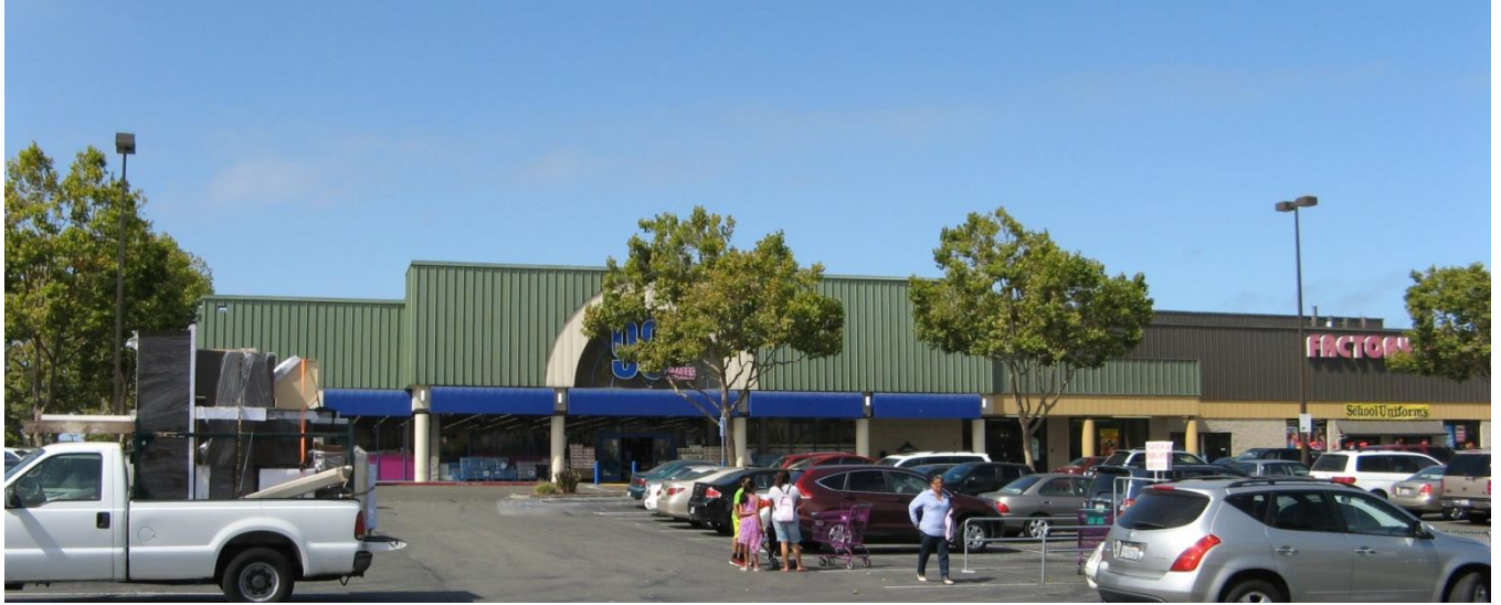
99 Cent Only and Factory 2 U, originally part of PD-83-3 and owned by Weingarten Realty Investments, but not included within the proposed project
