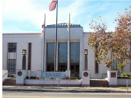
San Leandro City Hall
