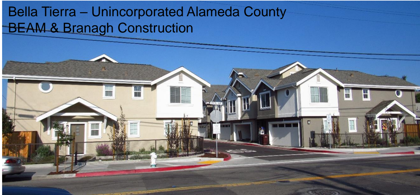
Ashland Place – Unincorporated Alameda County Branagh Construction
