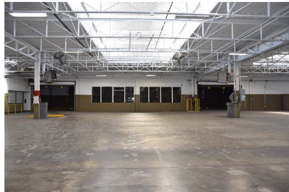
Picture 8: Warehouse interior, monitor roof above
