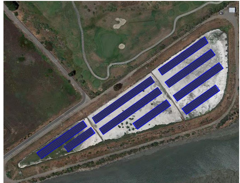
Water Pollution Control Plant
