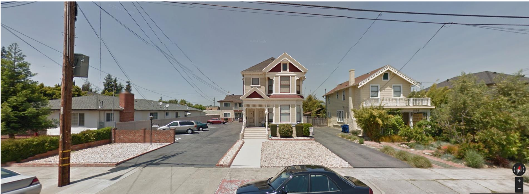
310 Warren Avenue (2011 street view, Historic – Victorian Residence; seven parcels west of the subject property)
