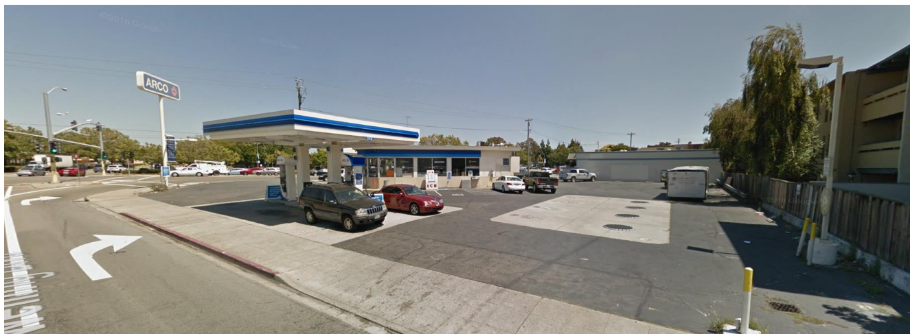
712 Lewelling Boulevard looking eastbound (Google 2016)
