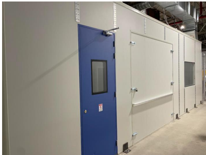
Figure 4 - Dry room exterior
