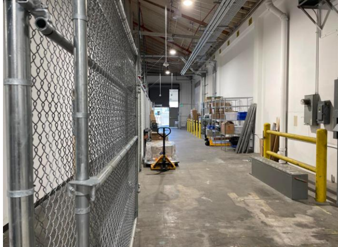
Figure 3 - Shipping and Receiving looking towards entrance
