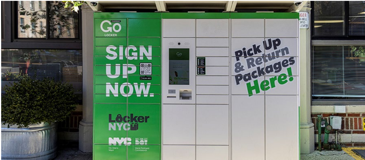
Centralized parcel delivery lockers, like this one from New York City Department of Transportation in Sunnyside, Queens, allow carrier services to consolidate deliveries at one convenient location for building tenants.
