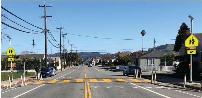
Rectangular Rapid Flashing Beacon
