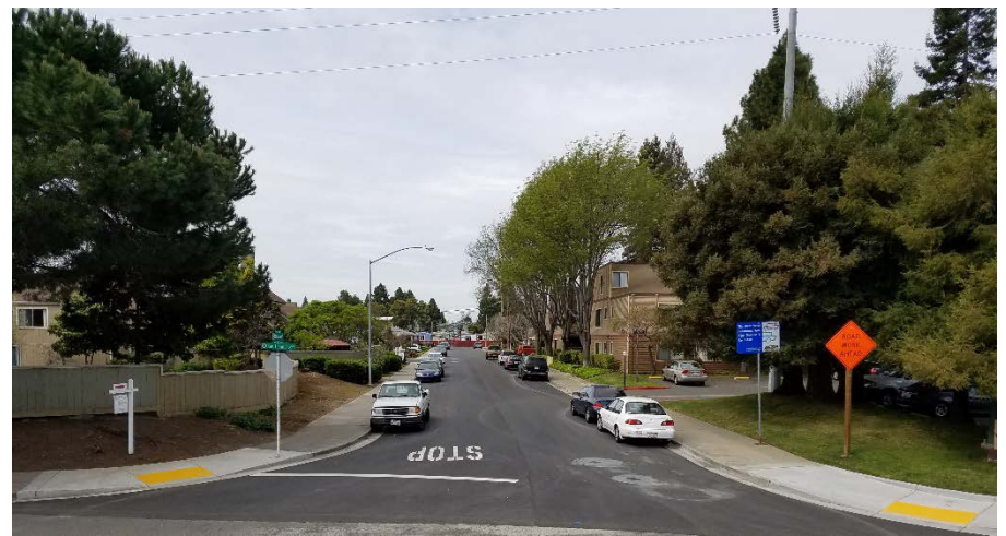
ROSE DRIVE (FULL DEPTH REHABILITATION)
