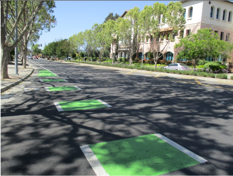
NEW PAVING ON SAN LEANDRO BOULEVARD
