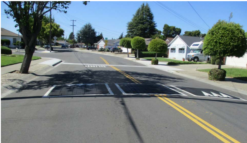
NEW PAVING ON EVERGREEN AVENUE
