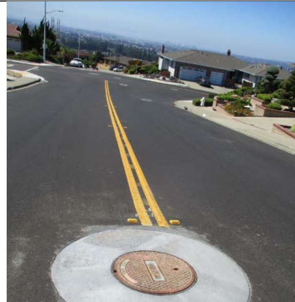
NEW PAVING ON MARINEVIEW DRIVE
