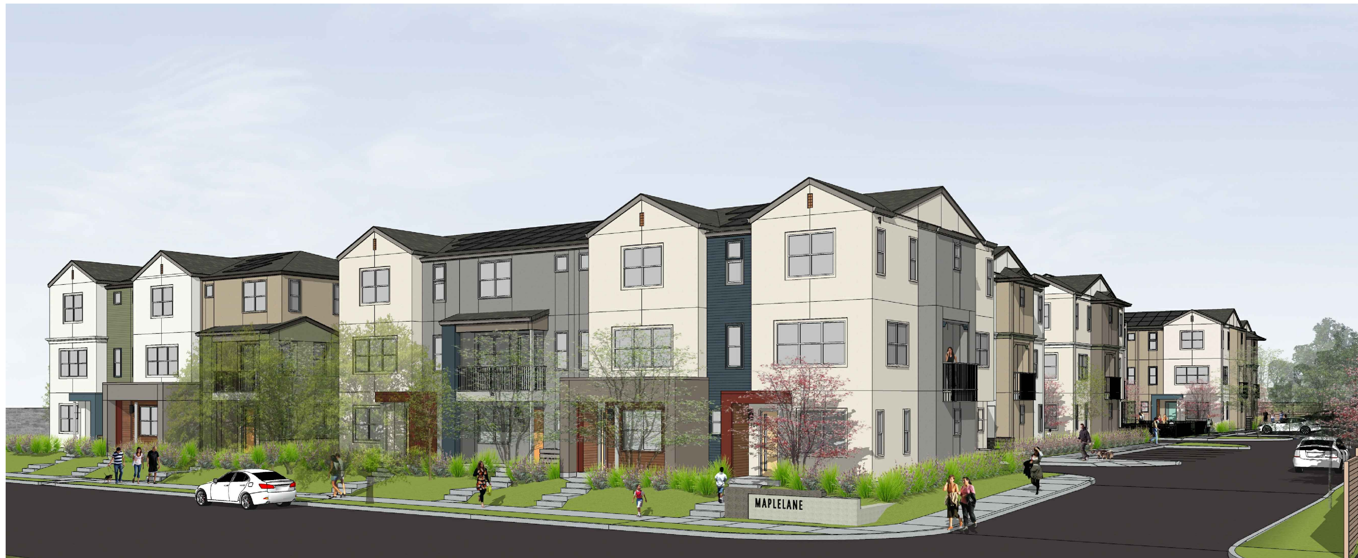
A - VIEW FROM ENTRANCE
