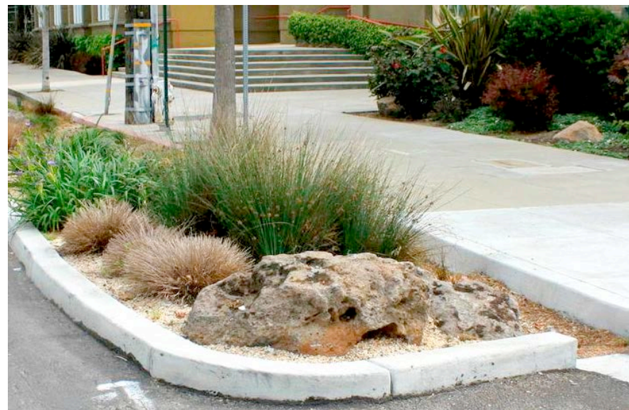
Rain garden removes pollutants in runoff using natural processes (Emeryville)
