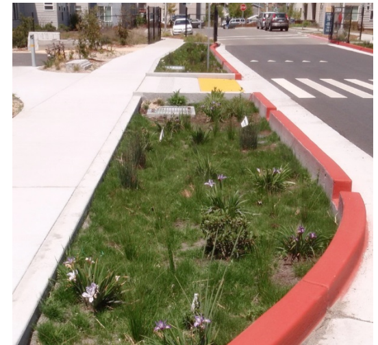
Bioretention area in Albany
