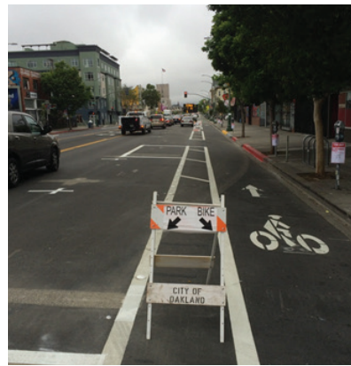
Example of one-way Class IV bikeway
