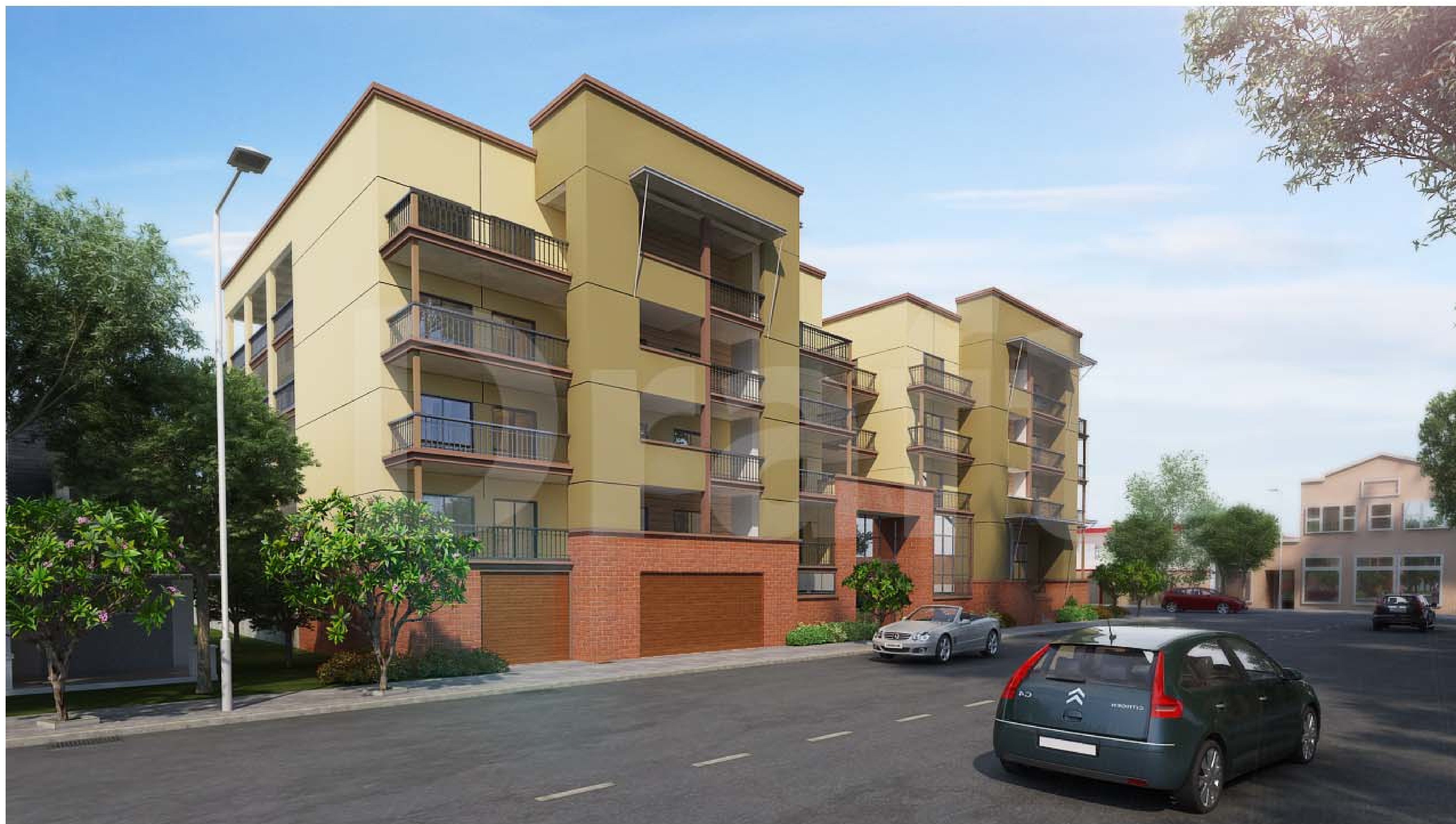
THE GALVAN BUILDING SOUTH ELEVATION WESTERN CORNER
