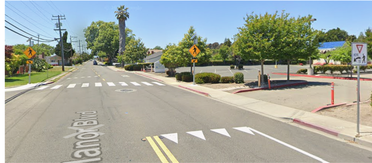
Example RRFB project at Manor Blvd and Grenda St
