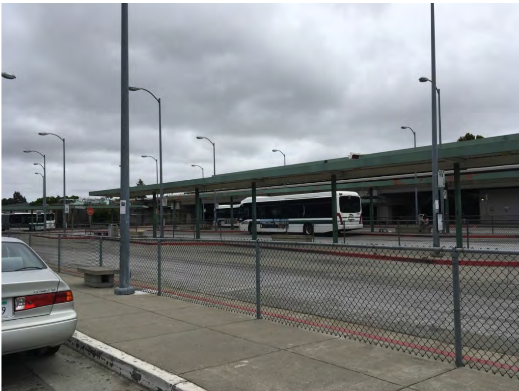
Figure 8f View of the Bay Fair BART Station
