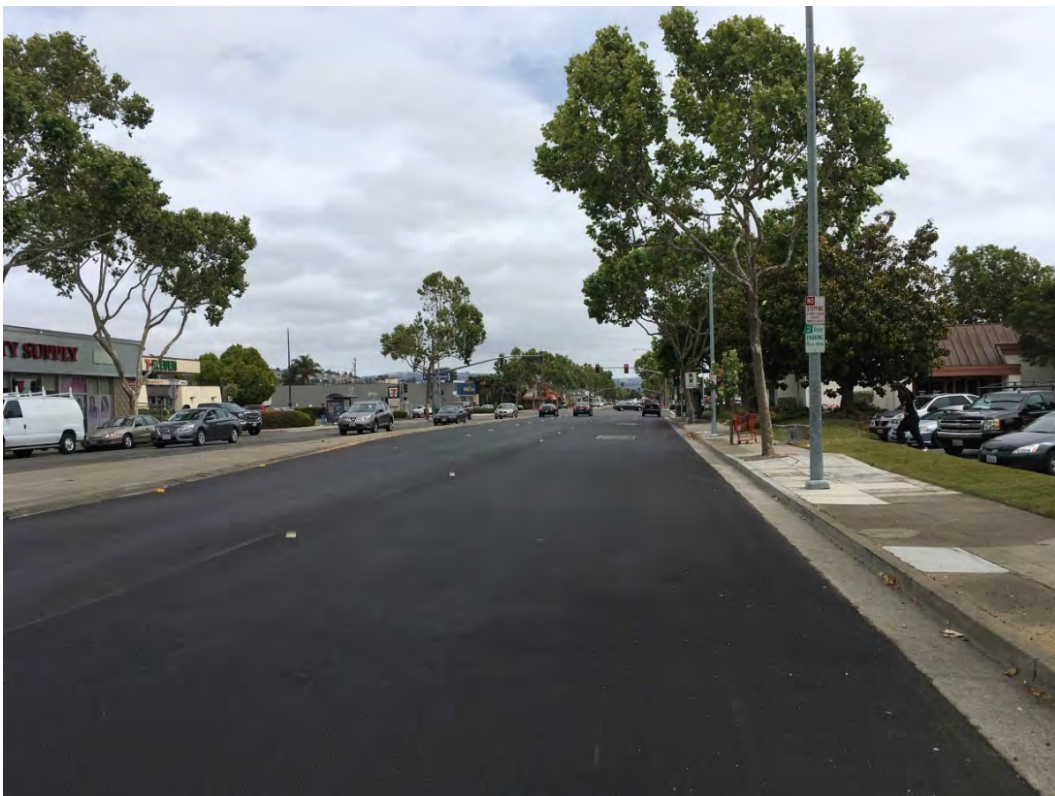
Figure 8h View Looking South along East 14th Street near 152nd Avenue
