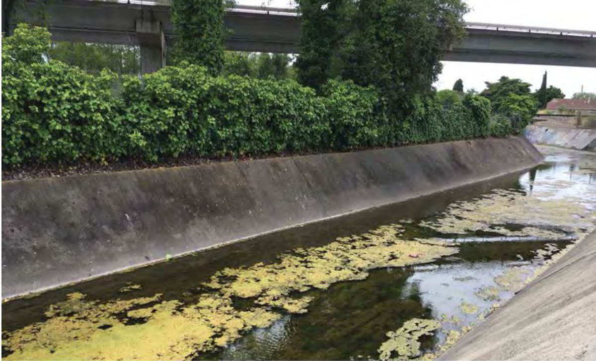
Photo 1: View of Estudillo Canal from Bayfair Center parking lot looking west.
