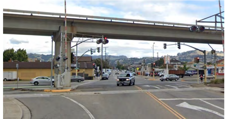
Vehicles at the intersection of Williams Street and San Leandro Boulevard
