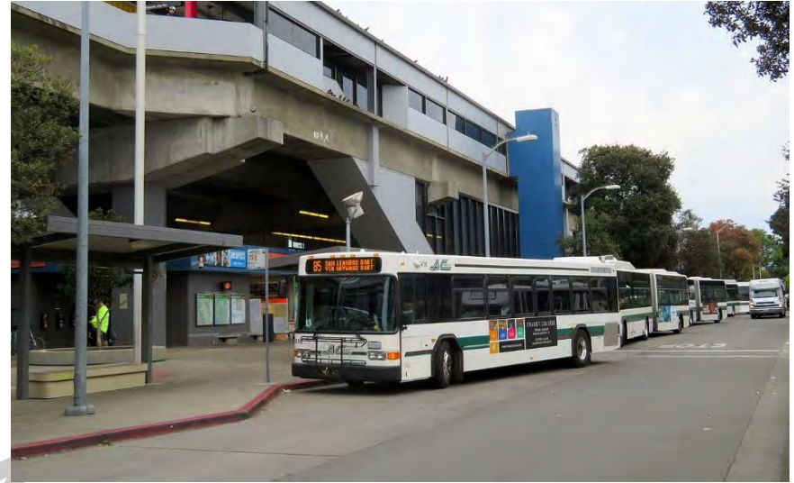
San Leandro BART Station
