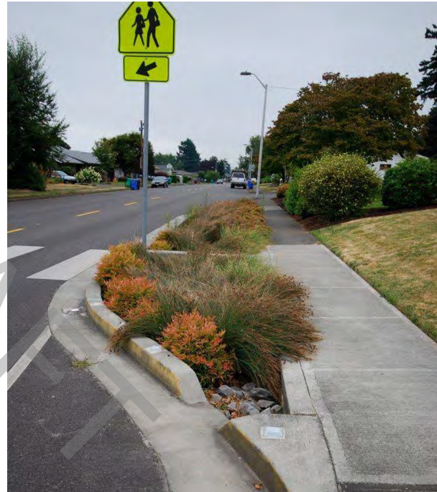
Example photo of a green stormwater bioswale in a pedestrian bulb-out. Plantings are low to ensure visibility of the crosswalk while greening the environment and providing stormwater recapture.
