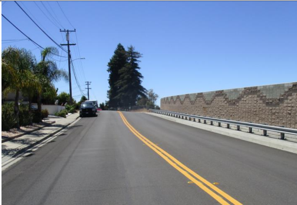
COMPLETED CAPE SEAL ON BENEDICT DRIVE
