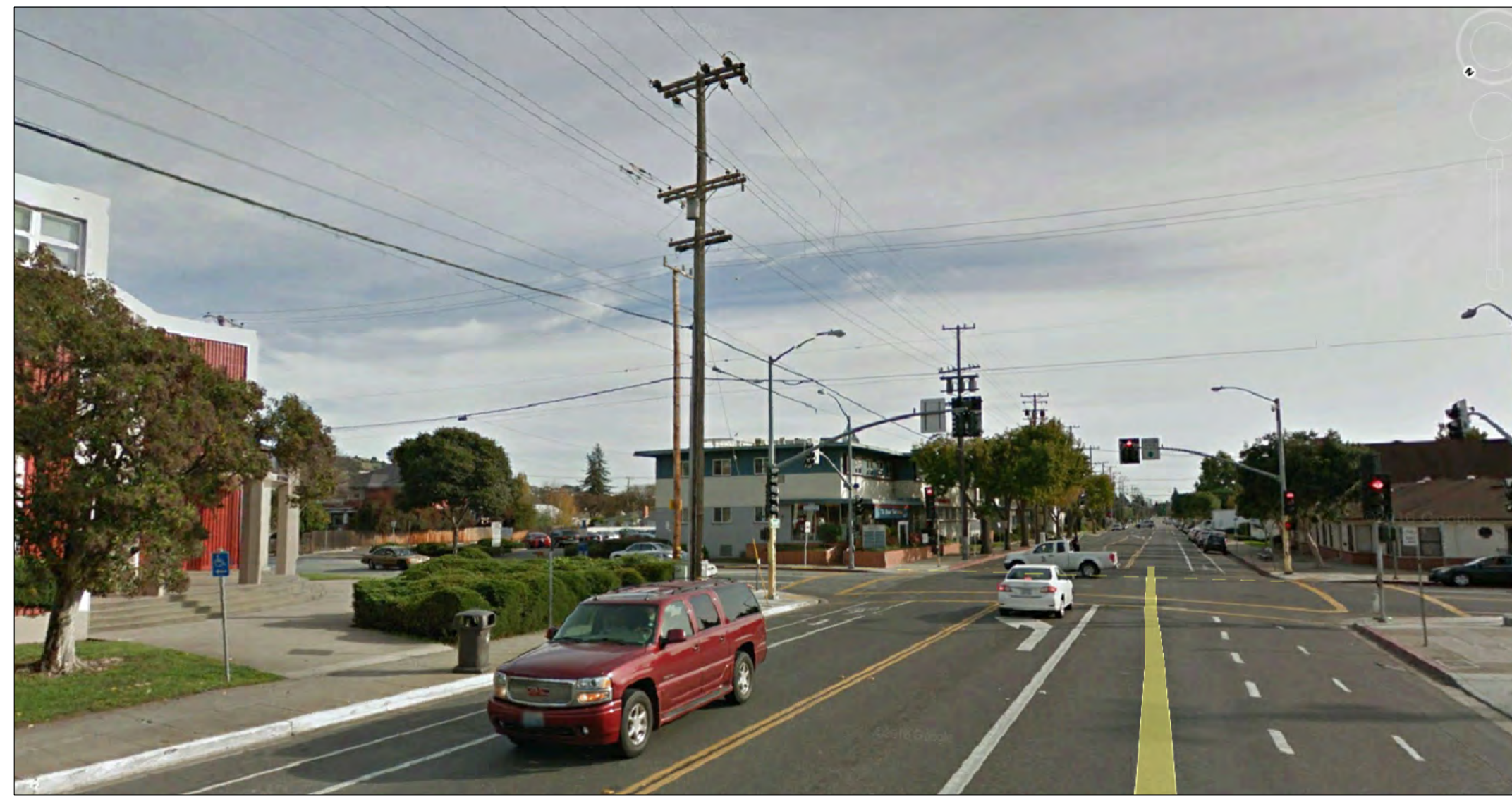
2 BANCROFT STREET LOOKING SOUTH
