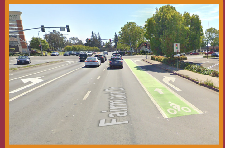
Green Thermoplastic Pavement Markings
