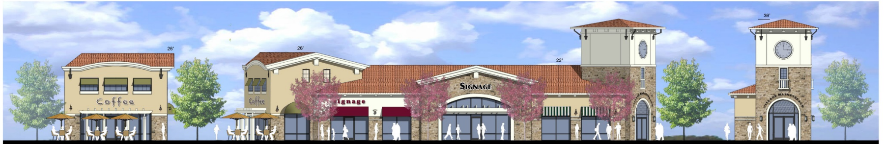
NORTHWEST AT CORNER
