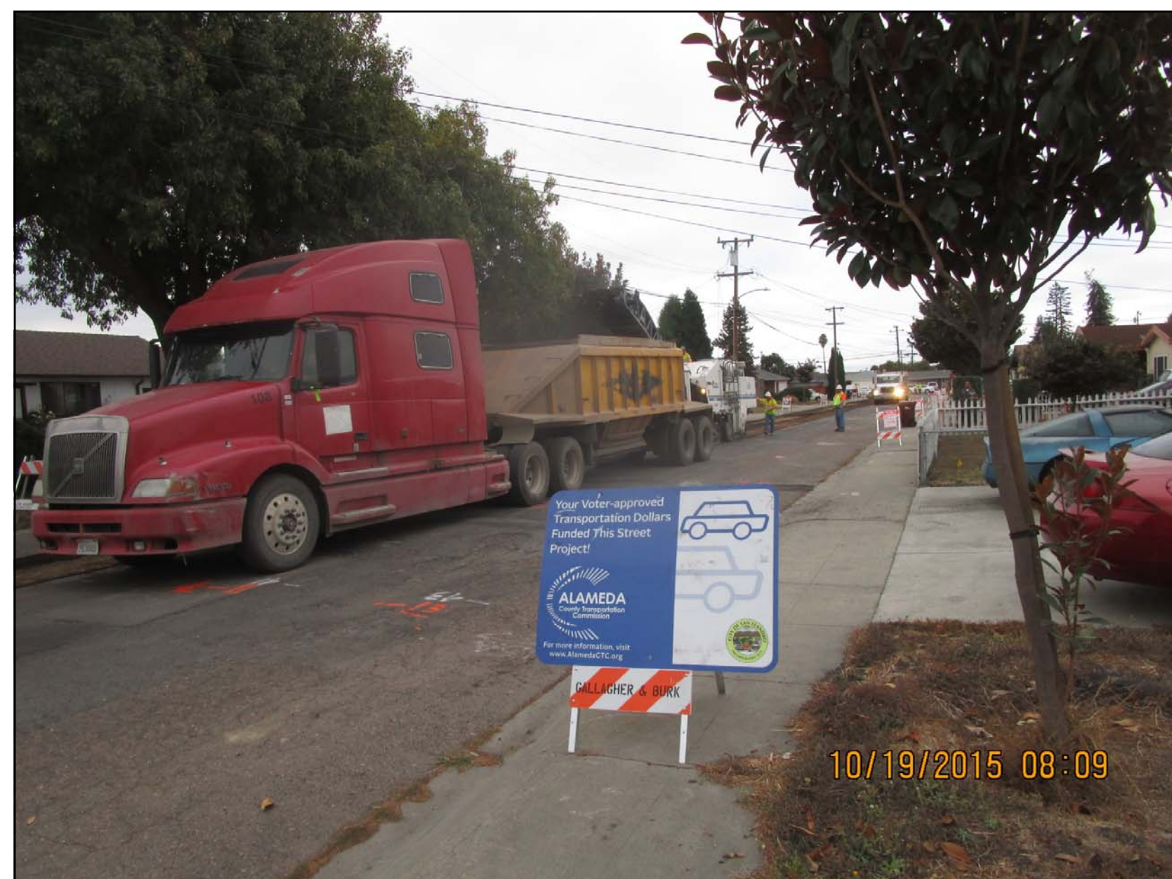
Grind and Remove Existing Paving
