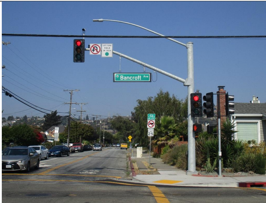
NEW SIGNAL AND NEW CURB RAMP, BANCROFT AVENUE
