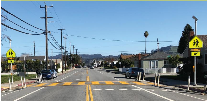
Rectangular Rapid Flashing Beacon
