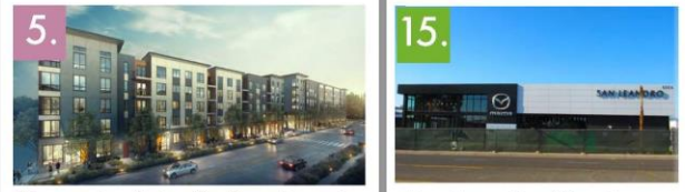
5. Alvarado-Antonio Apartments • 5.73 acre Transit Oriented Development • 687 residential units mix of studios, 1, 2, and 3 bedrooms 15. San Leandro Mazda 620 Marina Blvd. • New 122,000 sqft dealership and service center
