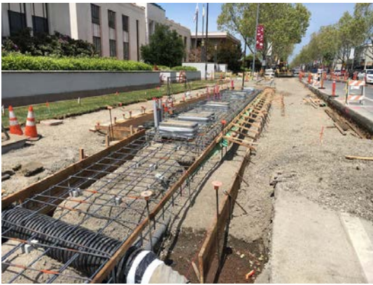
Civic Center Southbound Station
