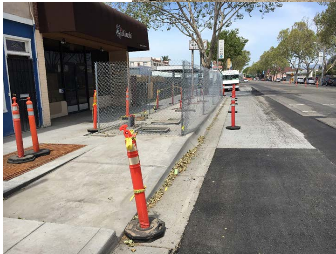
Georgia Way Southbound Station
