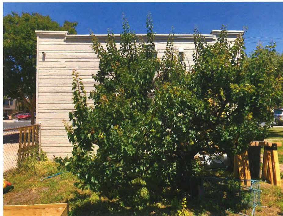
WEST ELEVATION AT REAR OF BUILDING
