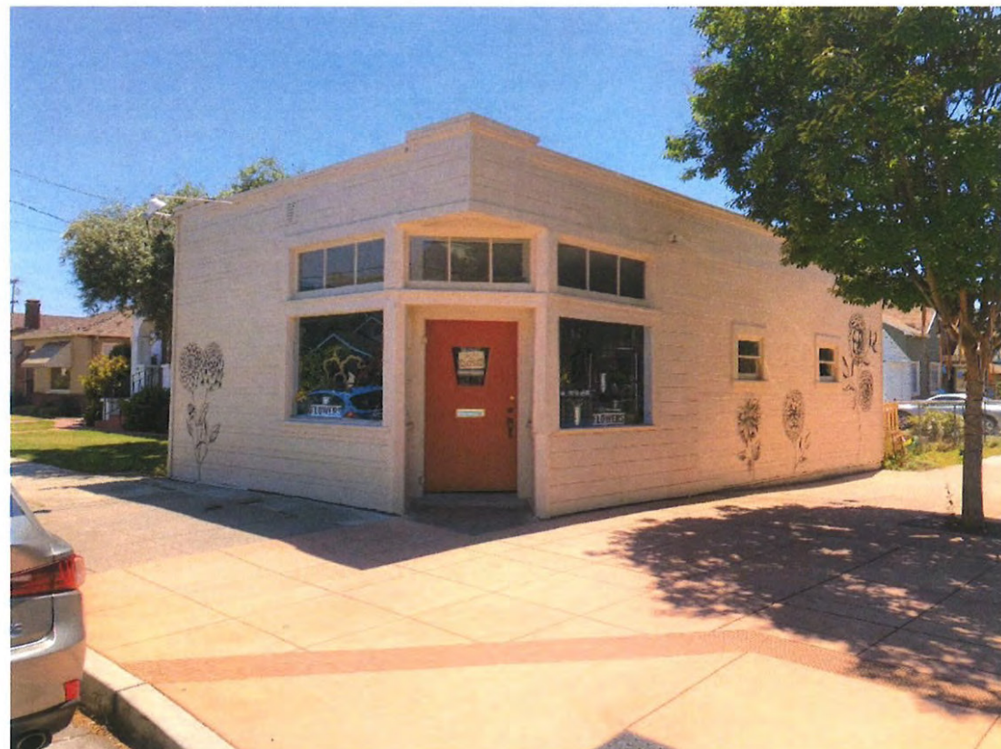
NORTH EAST CORNER VIEW
