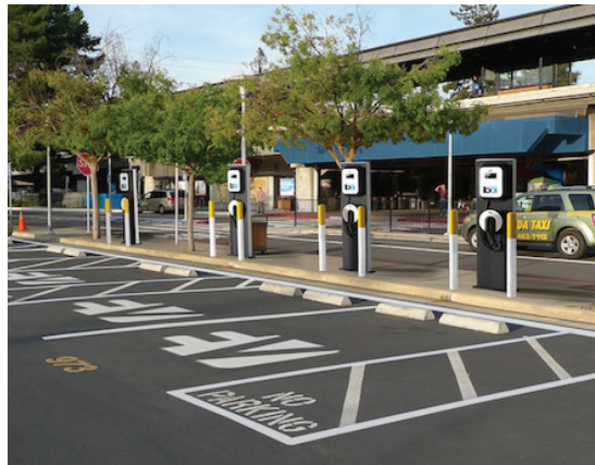
Example of electric vehicle charging station on BART parking lot
