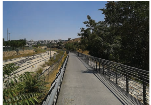
Example of an off-street path similar to the future East Bay Greenway
