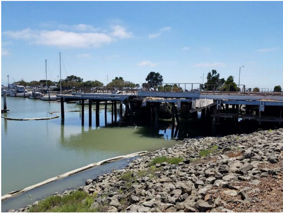
Photo 9 - Blue Dolphin Restaurant Foundation
