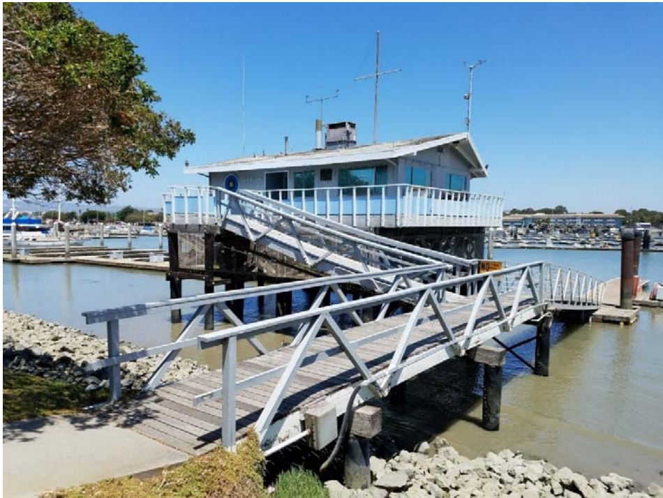
Photo 7 - Harbor Master's Office and timber access ramp
