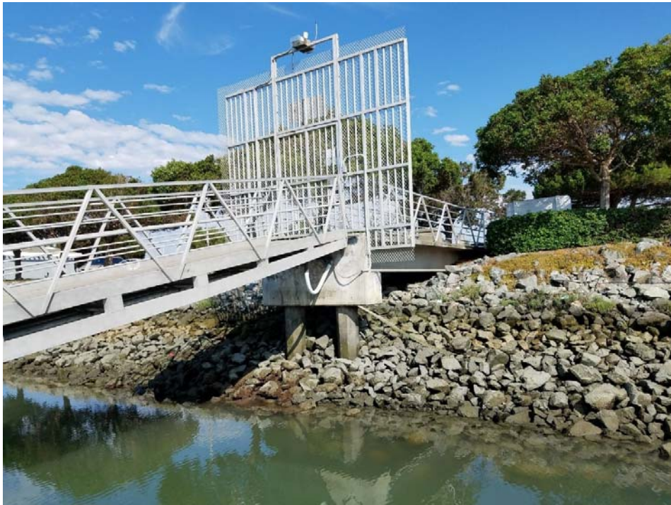
Photo 5 - Concrete Access Pier and Aluminum Gangway
