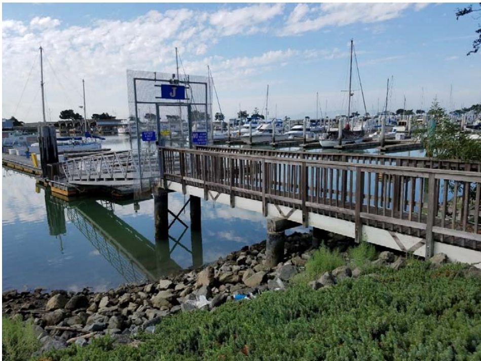
Photo 6 - Timber Access Pier and Aluminum Gangway
