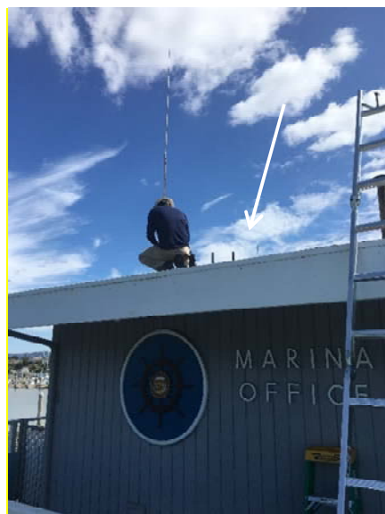
Photograph 5 – Marina – Harbor Master's Office – Roof – Roof Penetrations throughout (grey and black) (typical, indicated by white arrow) reported to contain asbestos.
