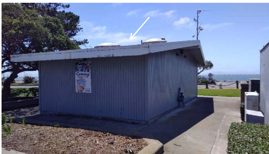
Photograph 1 – Marina – Restroom A, B – Roof penetrations – Penetrations throughout (indicated by white arrow) reported to contain asbestos.
