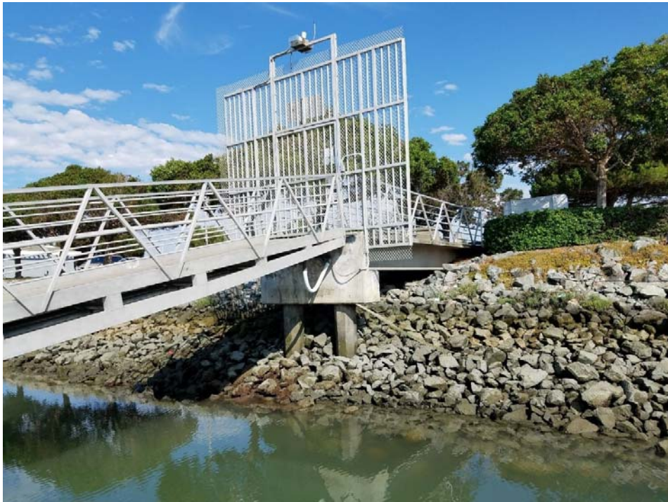
Photo 5 - Concrete Access Pier and Aluminum Gangway
