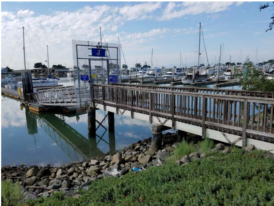
Photo 6 - Timber Access Pier and Aluminum Gangway
