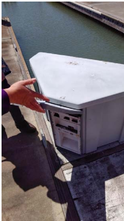
Photo 12 - Typical Service Cabinet – containing electrical, telecomm, and water service
