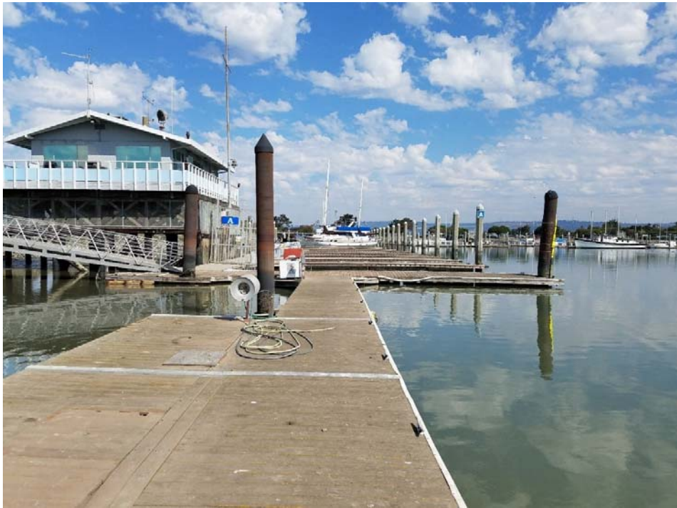
Photo 1 - Plastic lumber refueling dock with steel guide pile
