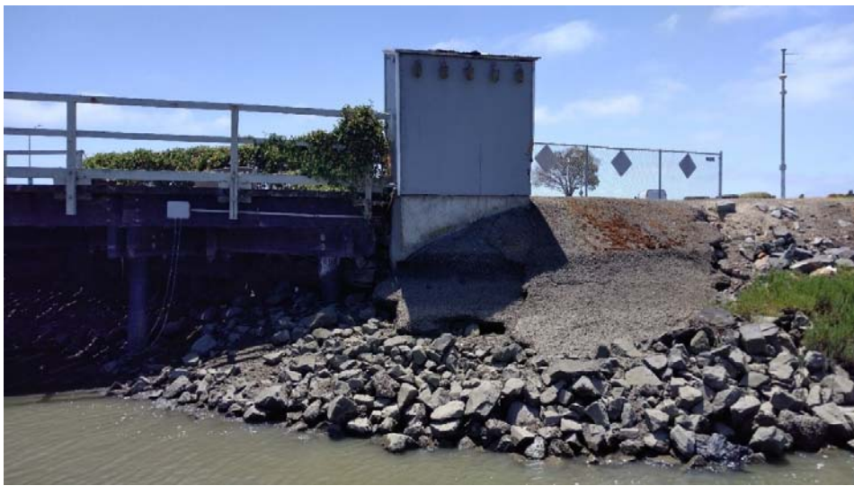
Photo 14 - Plywood Shed and Pile-Supported Closed Observation Deck
