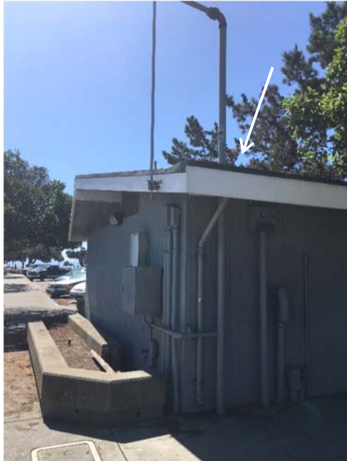
Photograph 6 – Marina – Restroom F – Roof – Roof Caulk (white/grey) (typical, indicated by white arrow) at penetrations throughout reported to contain asbestos.
