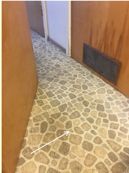
Photograph 4 – Marina – Harbor Master's Office – Resilient sheet flooring (tan/gold), 12"x12" vinyl floor tile (not shown, located underneath RSF) (indicated by white arrow) both reported to contain asbestos.
