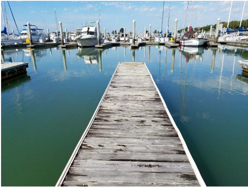
Photo 3 - Typical Condition of Timber Finger
