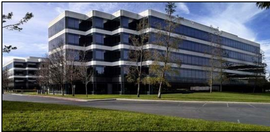
Current Buildings – Tenant Improvements
