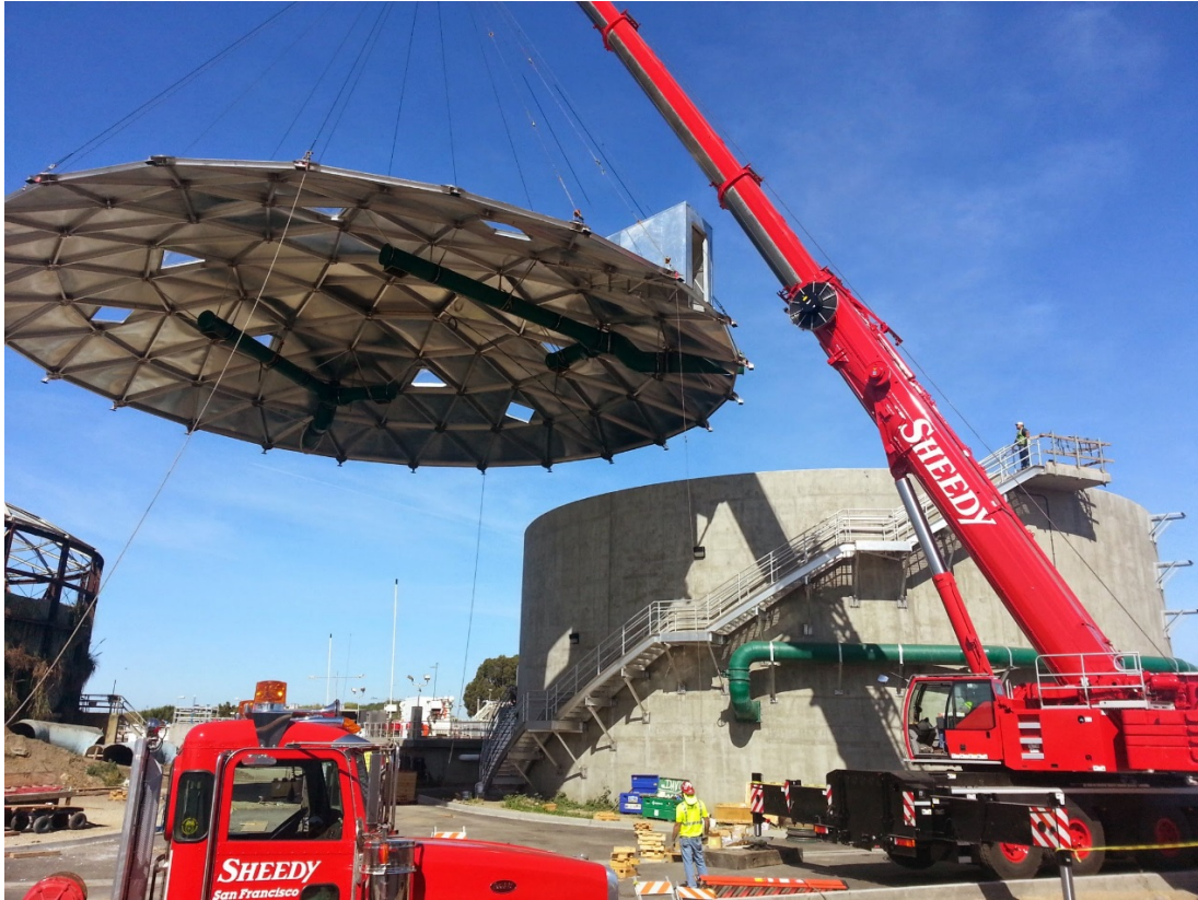
Construction of sewage treatment facilities
