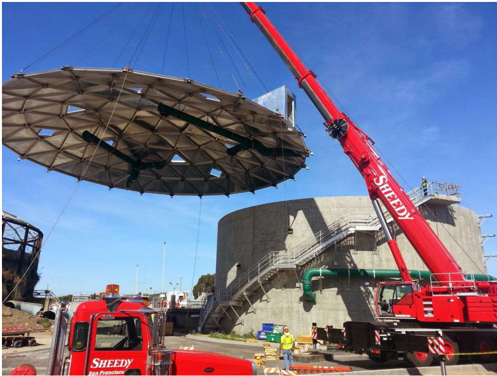
Installation of Trickling Filter Roof
