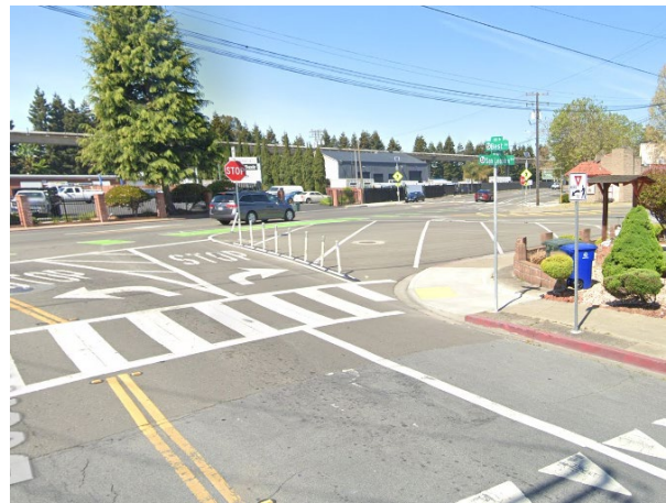
New curb extension to narrow the intersection, including accessible ramps and high-visibility crosswalks at San Leandro Boulevard and Best Avenue.
