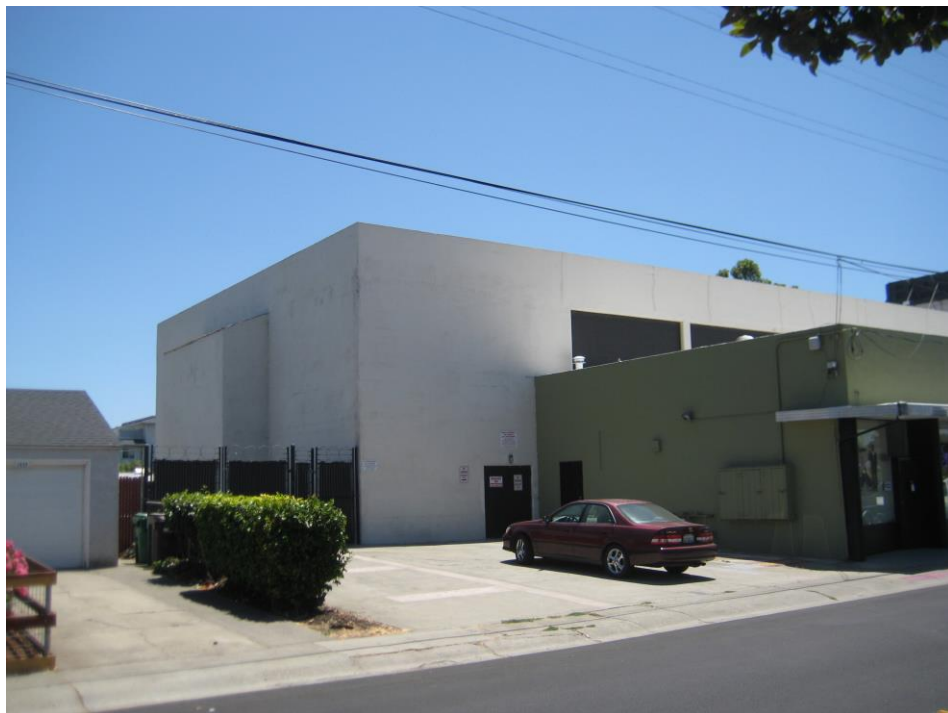
VIEW OF SIDE AND REAR FROM 148 TH AVENUE
