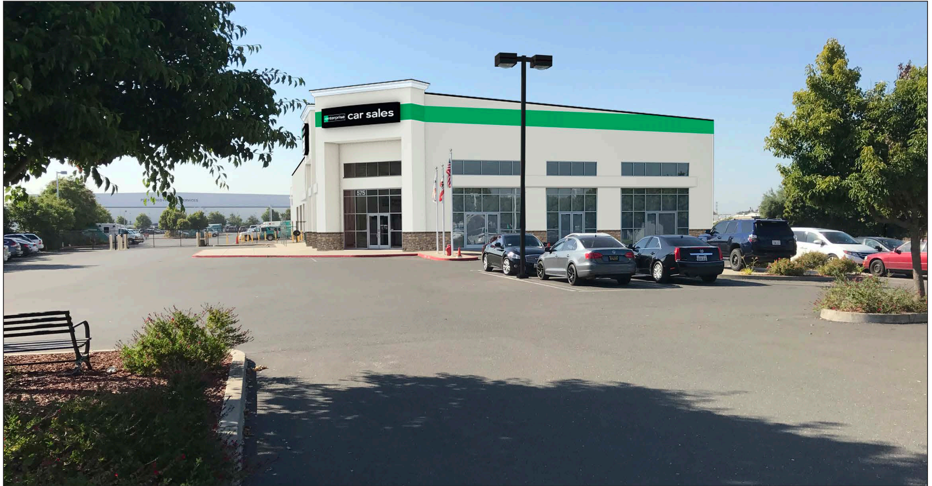
EXTERIOR | VIEW 1 | CAR SALES ILLUMINATED CABINET SIGN WITH PUSH-THROUGH LETTERING 4'-0"H X 20'-0"W
